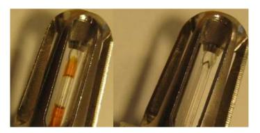
2.5.2. Sprinkler head with small air bubble that does not require replacement.
