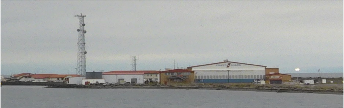
Port Angeles, WA – Air Station Port Angeles. Photograph by Randall Zempel
