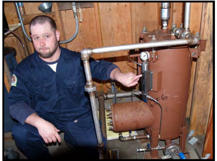
WG8 Shaun Fyfe pumps the hose fuel into the tank.
