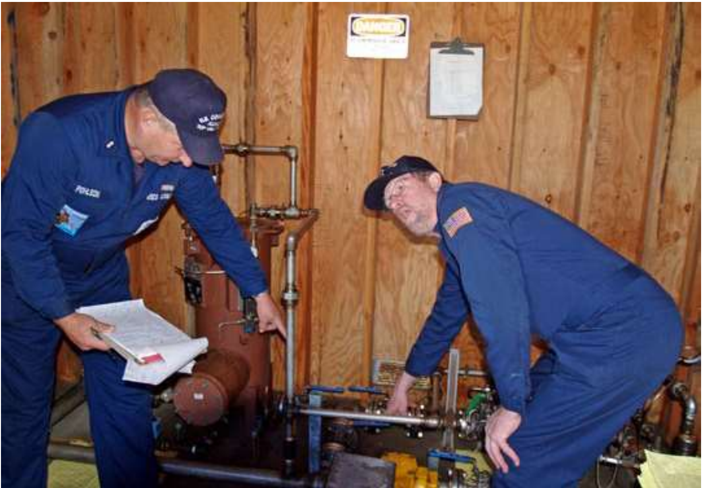
Doug Pohlson (left), FC-87, and Ken Reynoldson, FSO-CM 87 D11NR, identify the key valves in the fuel recirculation system.
