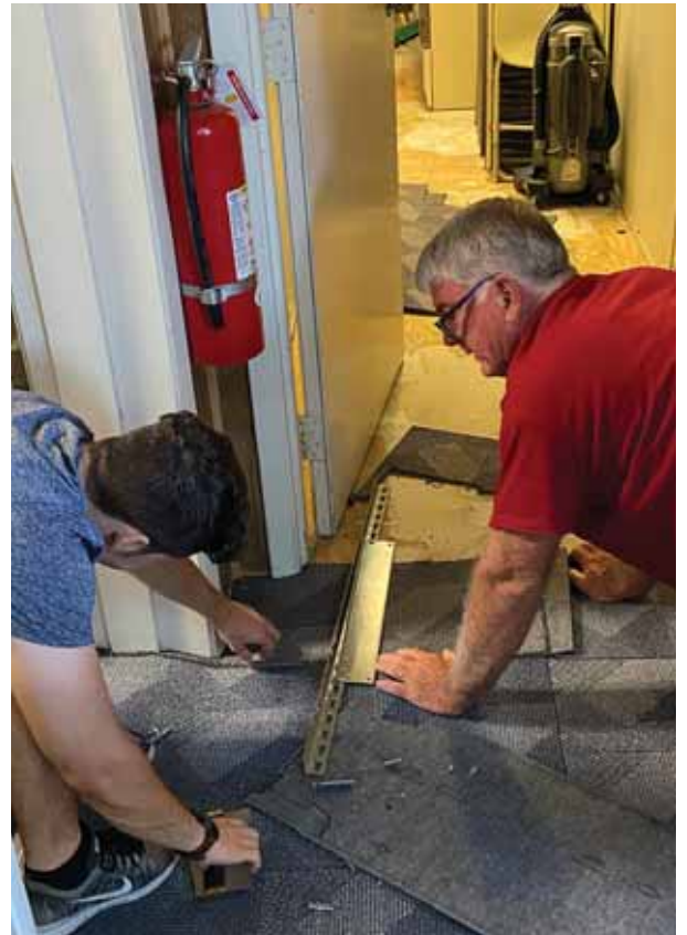
Tanner Piliego and Steve Williams complete installing the carpet tiles.
