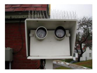
A new system is being implemented that is activated by the mariner's radio, called the Mariner Radio Activated Sound Signal (MRASS). This is similar to the system that pilots use to turn on runway lights at small airports.
