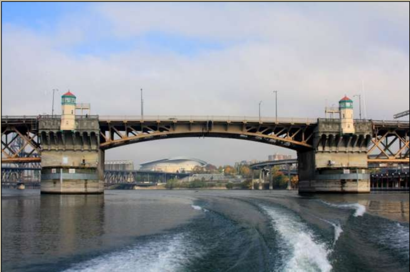
WILLAMETTE RIVER, Oregon—the Burnside Bridge in Portland, Oregon, in closed position. Photo by Auxiliarist Joann McCollum, Flotilla 78.
