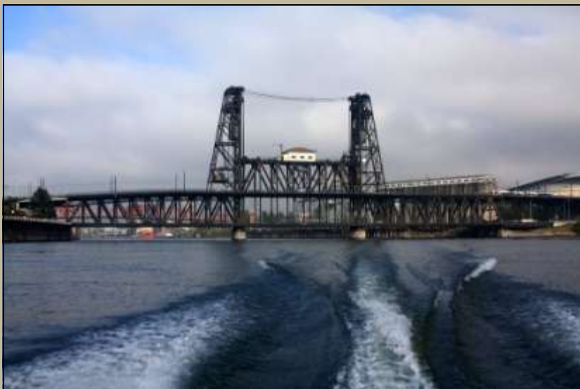
WILLAMETTE RIVER, Oregon—The Steel Bridge, a double deck lift bridge in Portland, Oregon, will deviate from its regular schedule on June 13, 2013. Photo by Auxiliarist Joann McCollum, Flotilla 78.
