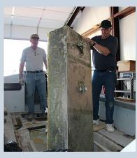
The old tank was removed and measured so that the new tank could be ordered. This tank holds seventy seven gallons of fuel and was common to Boston Whalers of that era.
