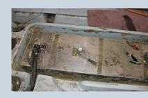
After several hours of foam removal Mike, John and Tom finally had all of the foam extracted. Fifty gallons of fuel also had to be siphoned from the tank which went smoothly. It was then time to remove this old tank!
