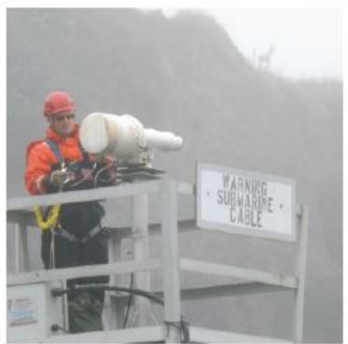
LCDR Twomey working on the Noyo River entrance range light.
