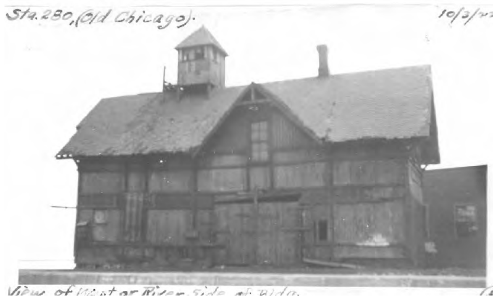
Original photo caption: "View of West or River side of Bldg. [;] Sta. 280 (Old Chicago)." Photo dated 3 October 1922.
