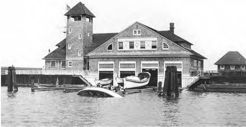
Original photo caption: "U.S. Coast Guard Station No. 280 [;] Illinois-Central Pier No. 1 [;] Chicago, Illinois." No date indicated. Photo taken by "Special Service Co. Photographers of Austin, Ill." Note the crew practicing their capsizing drill with the station's lifeboat.
