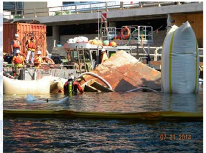
The barge is brought to the surface. Diver in the foreground attached connections for pumps and high-pressure air to float the barge. Supplemental lifting bags are also visible.
