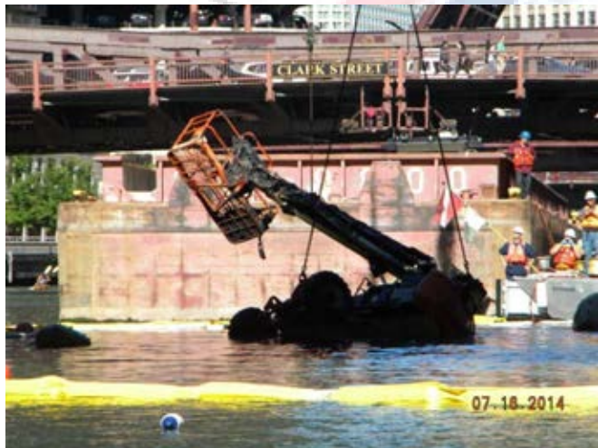
A man-lift is raised off the sunken barge. We were assured this would mean the salvage would be completed in one more day. No such luck!
