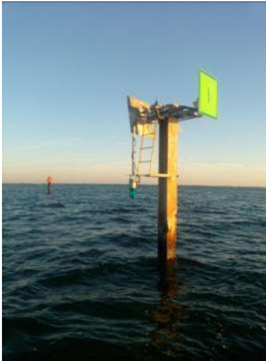
Damaged Light 1 at the river entrance to the Pithlachascotee River.
