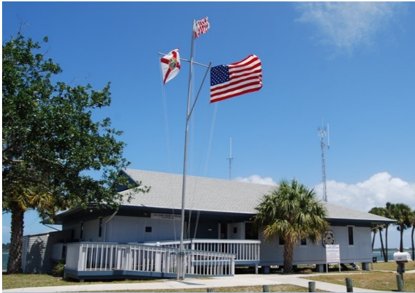
Flotilla 59 Headquarters Building Sandsprit Park, Martin County.
